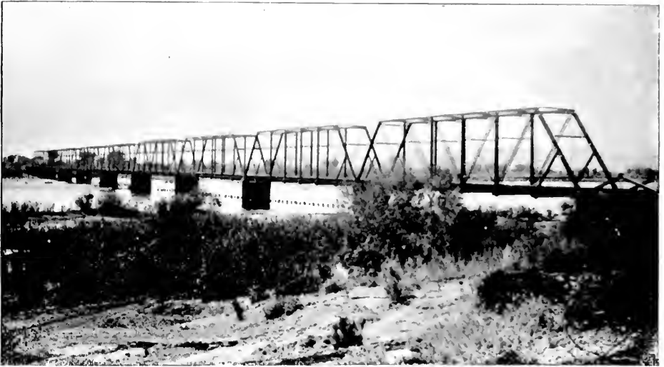
Maricopa and Phoenix Railroad Bridge
